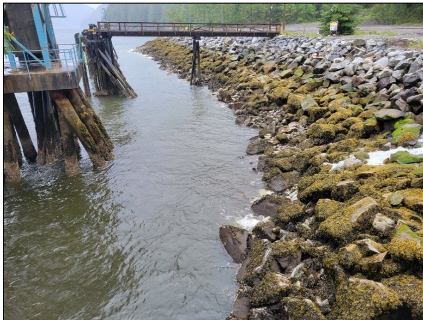
Photograph 8: Shoreline between the west barge landing and the Ro-Ro. Riprap with green algae and rockweed bands visible.
