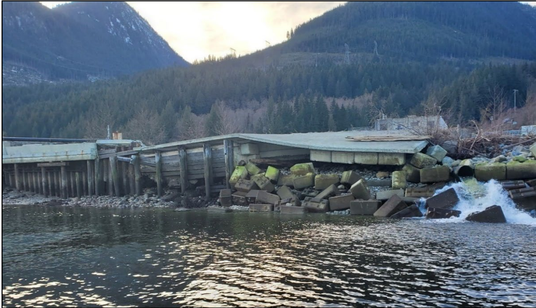
Photograph 7: Remnants of an old timber wharf and an outfall east of Mill Creek. The timber wharf makes up most of the intertidal zone in this section, with natural cobble, gravel and sand near the low water line.
