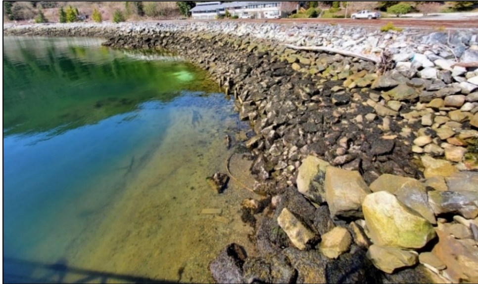
Photograph 5: Looking west at the shoreline between the access dock and Ro-Ro showing the transition from riprap with rockweed to bare silty sand, gravel, and sparse cobble in the subtidal zone with some wood debris.
