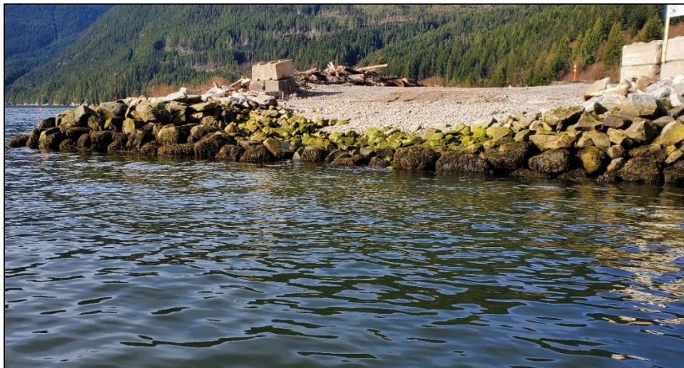
Photograph 16: Typical backshore conditions at the east barge landing. Generally highly disturbed, former industrial areas with gravel, concrete, riprap or cobble and no vegetation. Green algae and rockweed bands are visible on riprap armoured sections of the shoreline.
