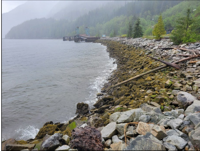
Photograph 9: Riprap armoured shoreline east of the Ro-Ro with green algae and rockweed bands typical of armoured slopes throughout the site.
